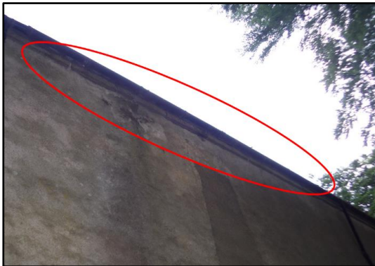
Photo 1: Example of deteriorating masonry at wall head and under guttering.
